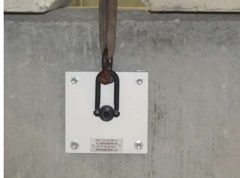
PLATE PICK POINT INSTALLED
